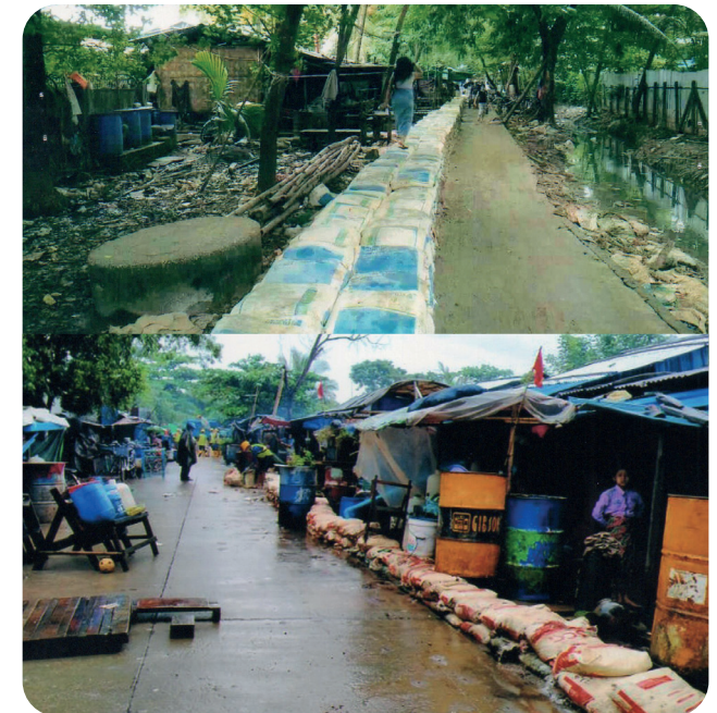
Flood protection by sandbags in North Okkalapa and Dagon Myothit (South) Townships Photo: Drainage and Sewerage Management Department
