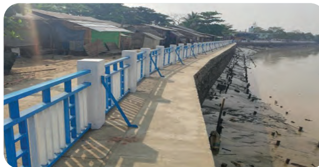
Flood protection by retaining wall in Dagon Myothit (North) Township Photo: Department of Water Resources and Rivers Development
