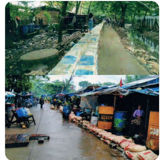
Flood protection by sandbags in North Okkalapa and Dagon Myothit (South) Townships Photo: Drainage and Sewerage Management Department
